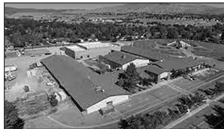
The newly renovated Swope Middle School held its grand re-opening on Jan. 30 after 14 months of work.
